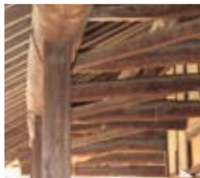
Firm-fitting timber joinery in the storehouse
