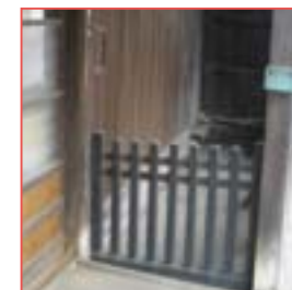
Low latticework fence ( komayose ) used to prevent horses and porters from gaining access.
